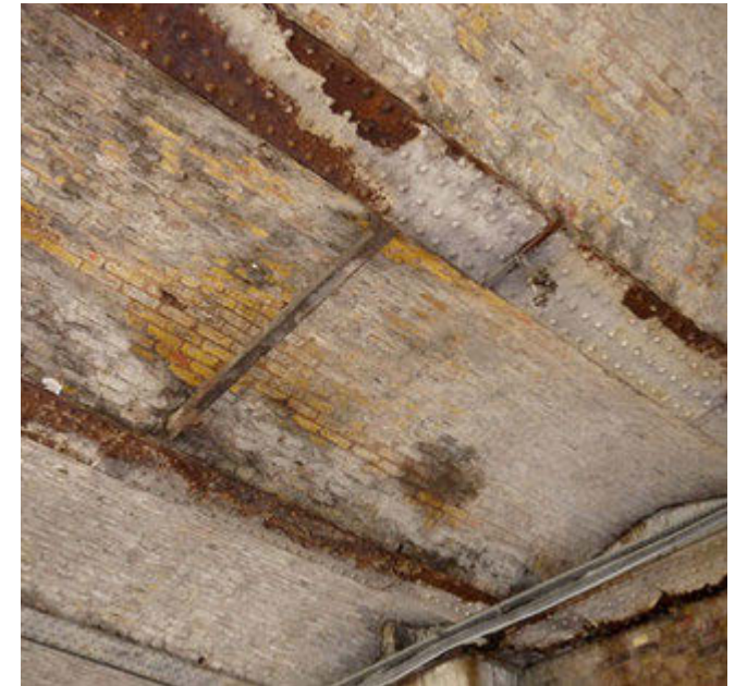
Fig 6.3.56: Poor condition steel work, jack arches (clockwise from above)
