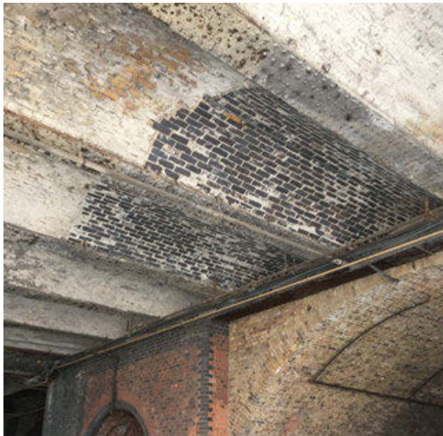
Fig 6.3.55: London Road jack arches, as existing
