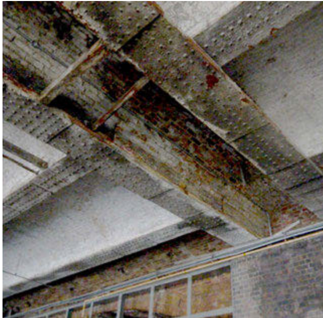
Fig 6.3.56: Poor condition steel work, jack arches (clockwise from above)
